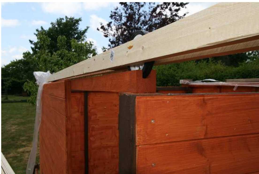
Figure 36 – Checking roof runner wheels for free motion in side runners
