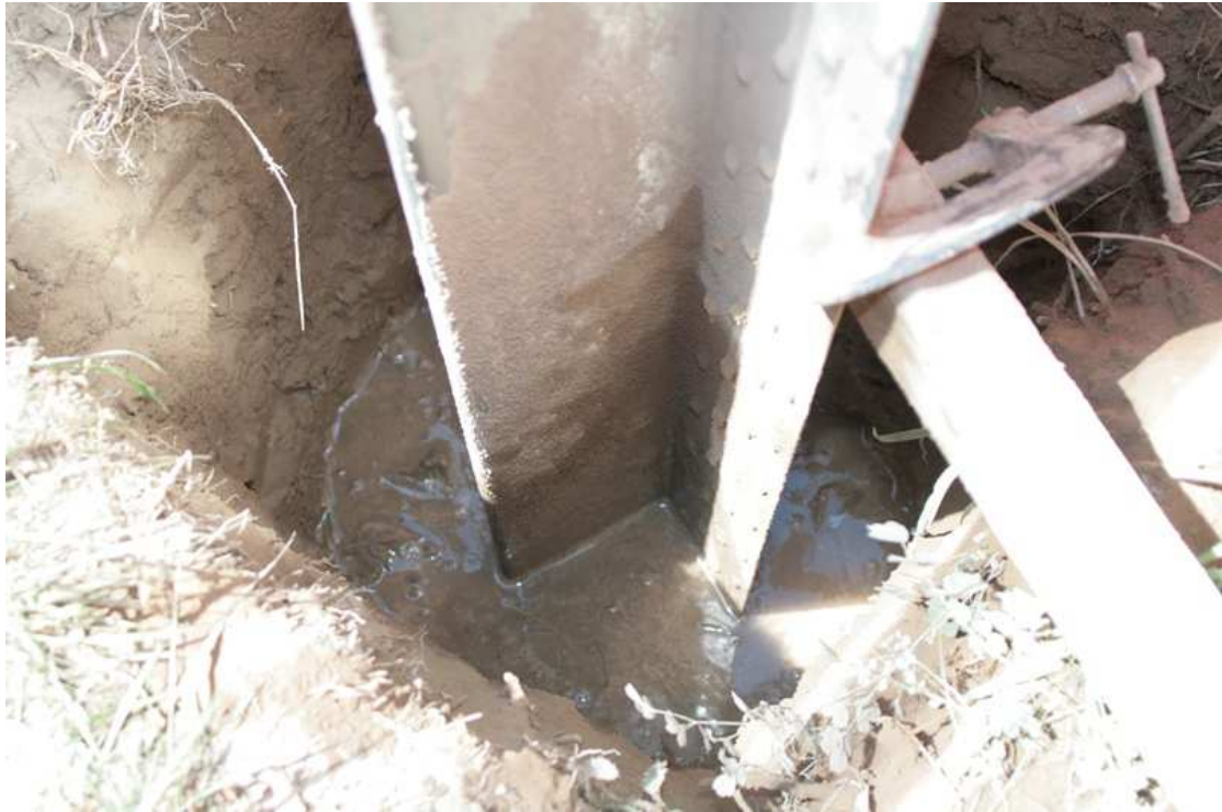
Figure 64 – Concreting the Lintel into the ground
