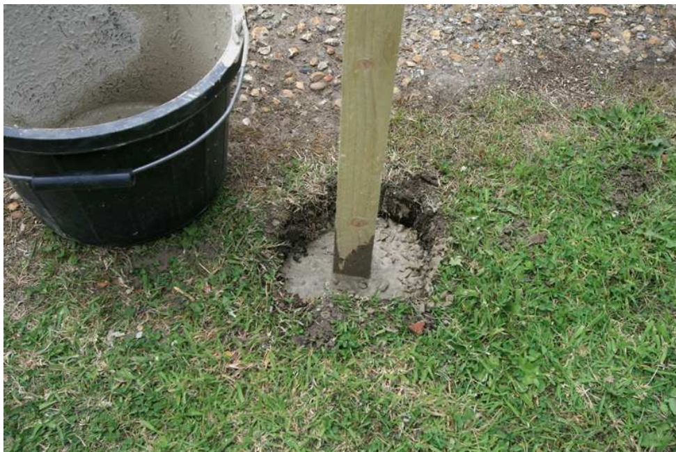
Figure 74 – Roof runner supports posts concreted into ground
