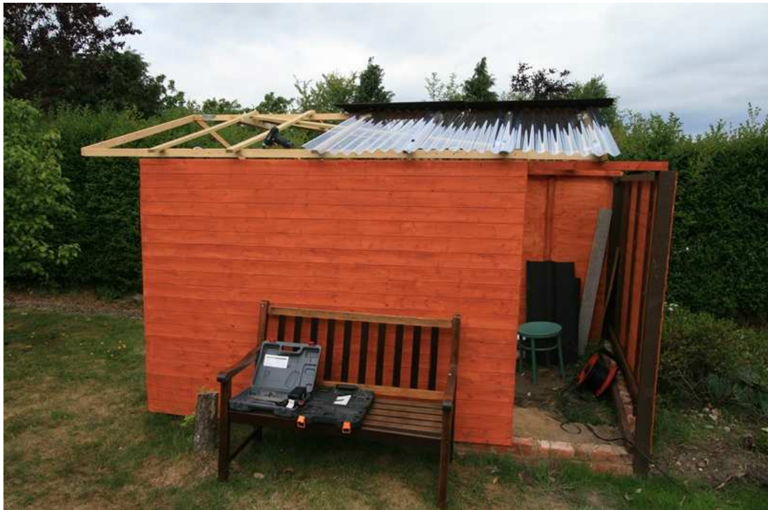
Figure 54 – Adding the plastic corrugated sheets and roof ridge (1)
