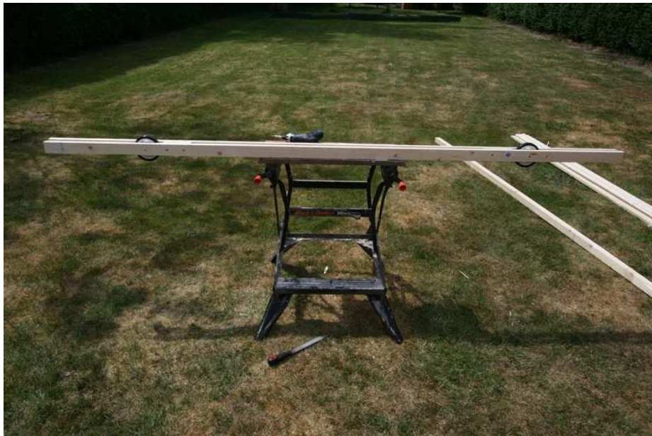
Figure 33 – A roof runner with its two captive wheels in place
