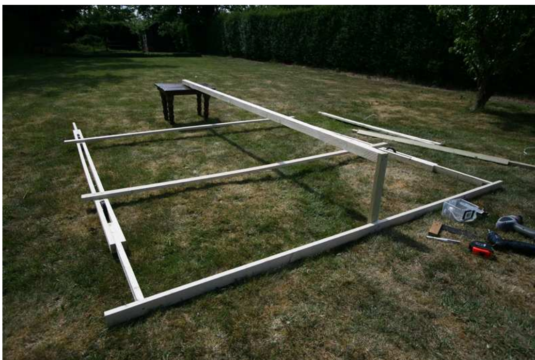
Figure 41 – Roof assembly in progress (temporary cross braces also visible)
