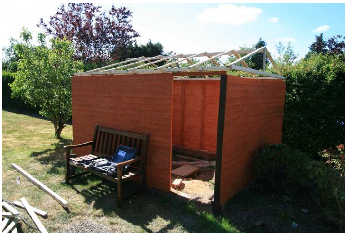
Figure 45 – Roof placed into position (1)
