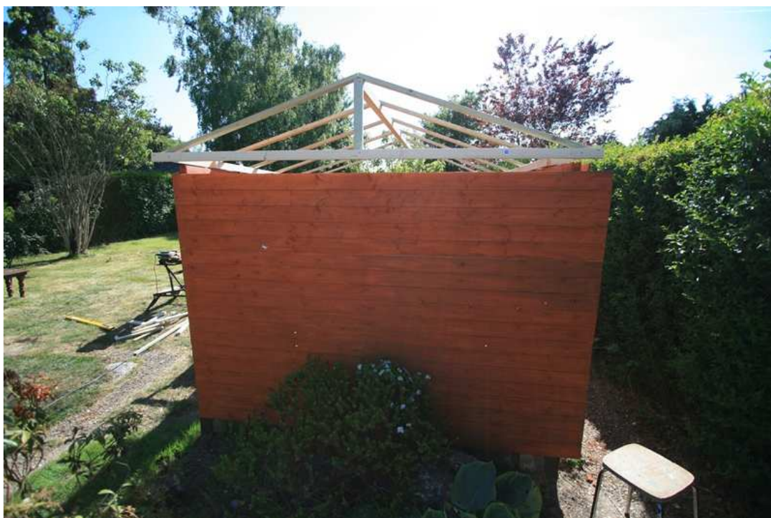
Figure 48 - Roof placed into position (4)
