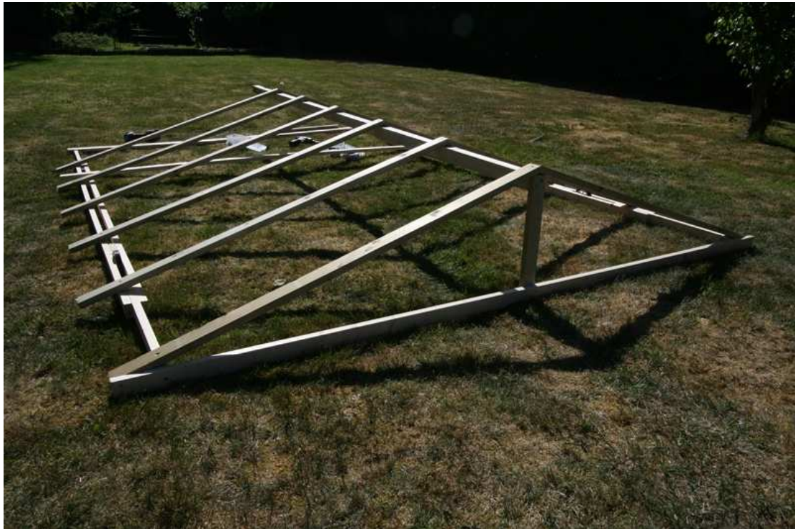
Figure 31 – The completed roof frame
