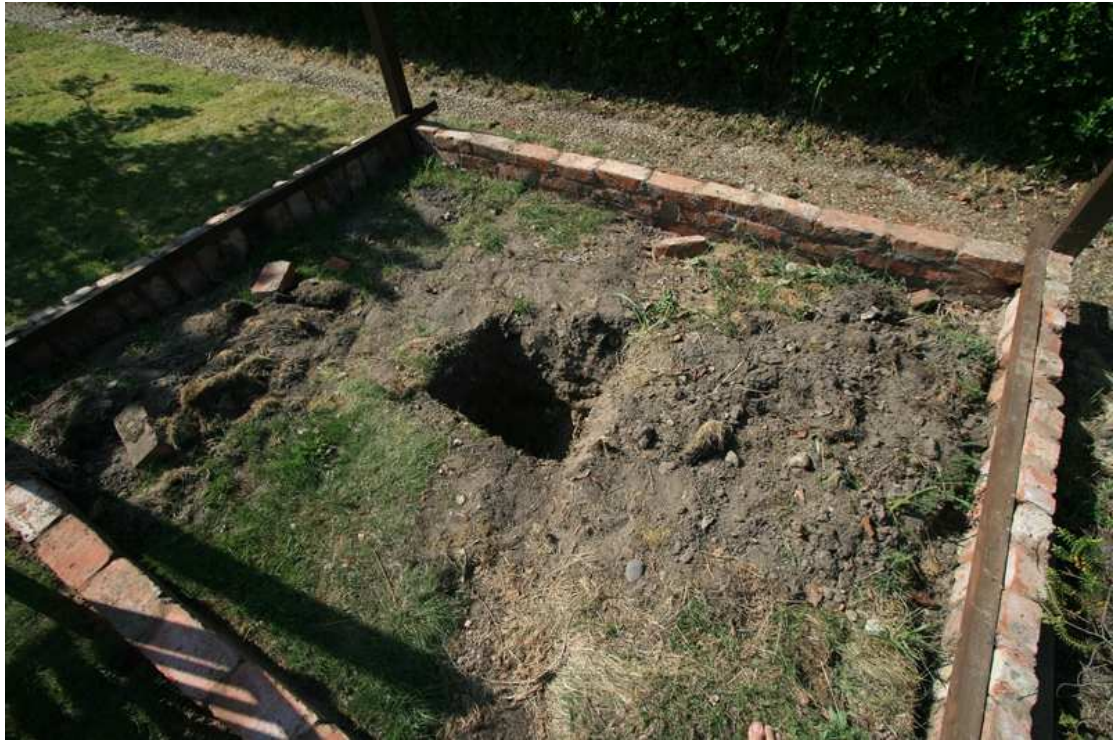
Figure 15 – Brick base completed (1m deep hole for pier also visible)
