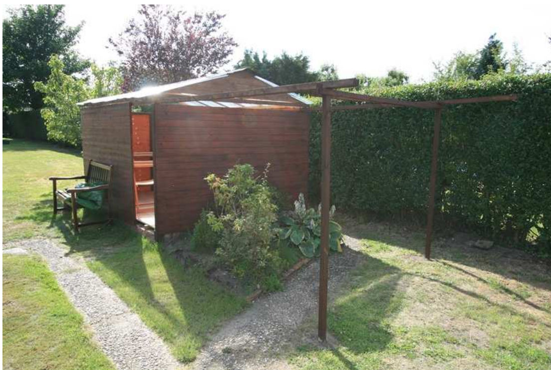
Figure 75 – Roof runner supports in place
