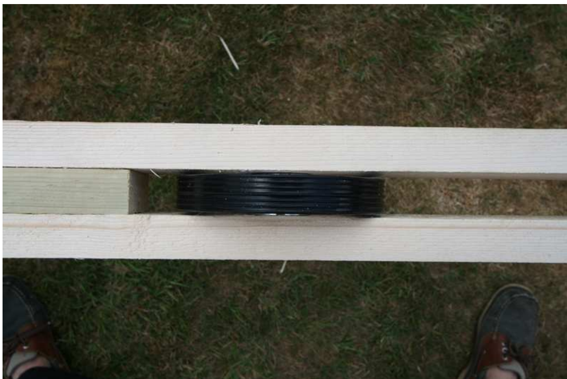
Figure 35 – Another close up of captive roof runner wheel
