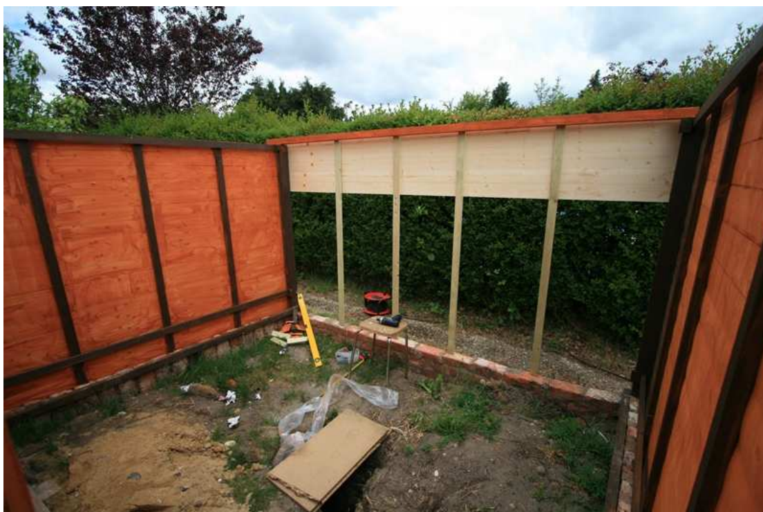
Figure 27 – Last side in progress – with other roof runner in place
