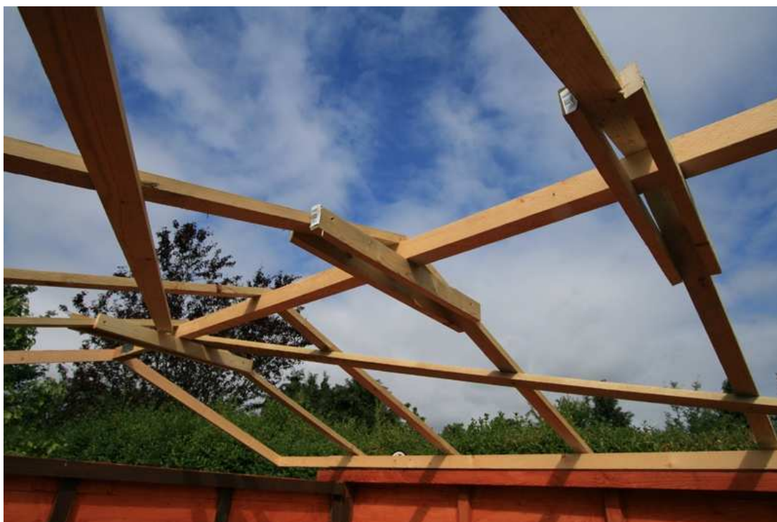
Figure 52 – Adding roof cross braces and brackets (2)
