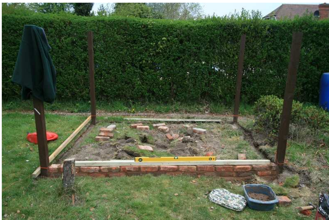
Figure 13 – Laying the two levels of brick
