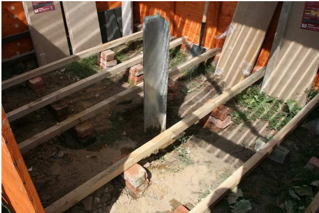
Figure 65 – Add beams for floor support
