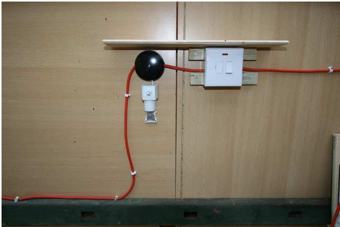
Figure 86 – Main feed into fused switch
