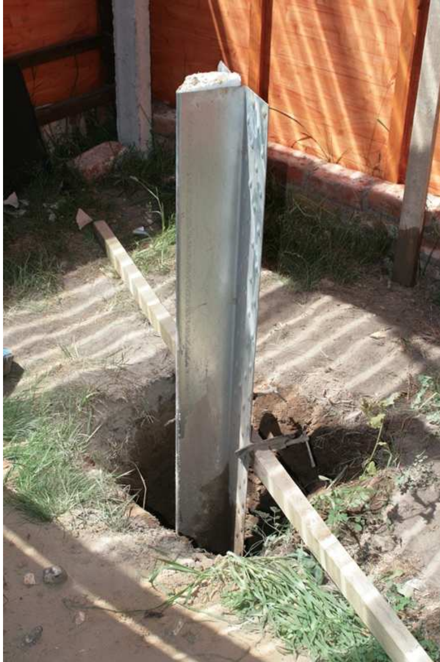
Figure 63 – Positioning the Pier
