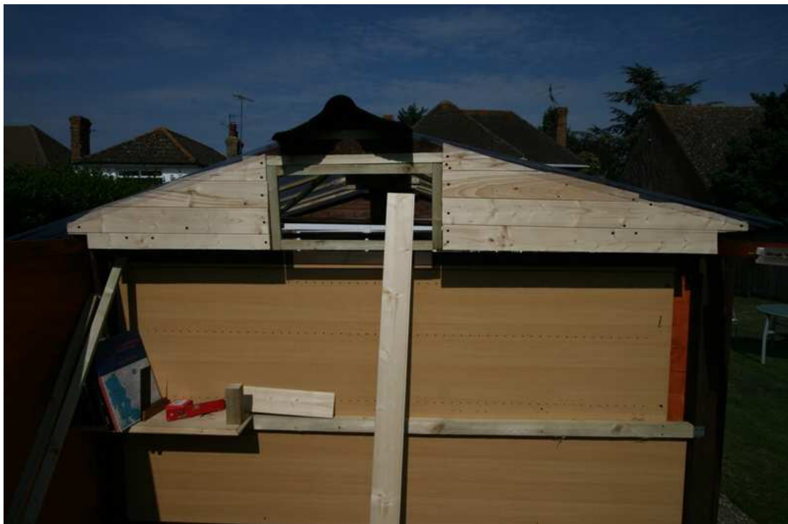
Figure 61 – Roof end with scope clearance door in progress
