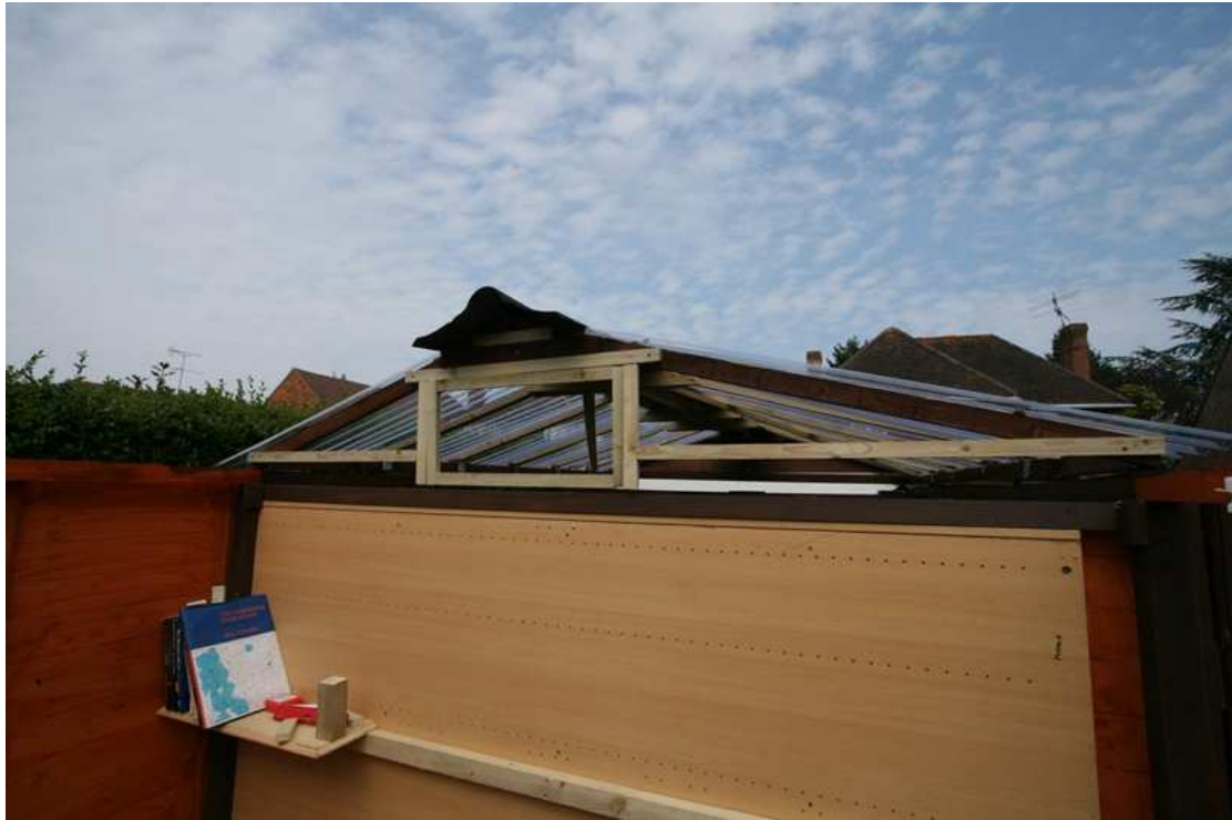
Figure 60 – Add one roof end with a hinged door to allow for scope clearance
