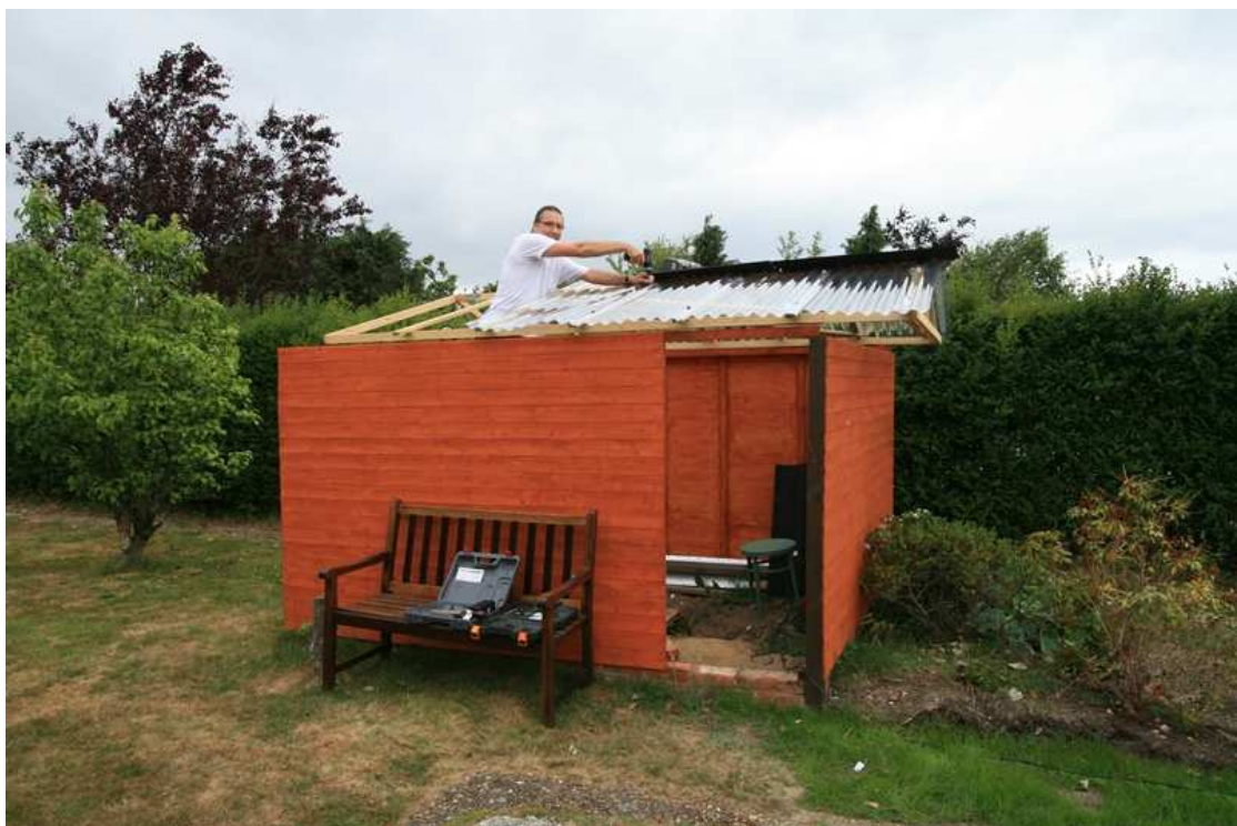
Figure 55 – Adding the corrugated plastic sheets and roof ridge (2)
