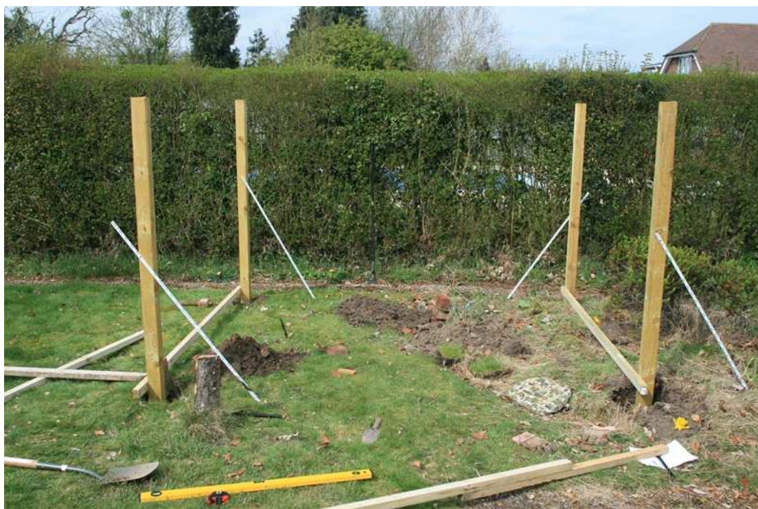
Figure 8 – Ensure the corner posts are equal spaced, level and square to each other
