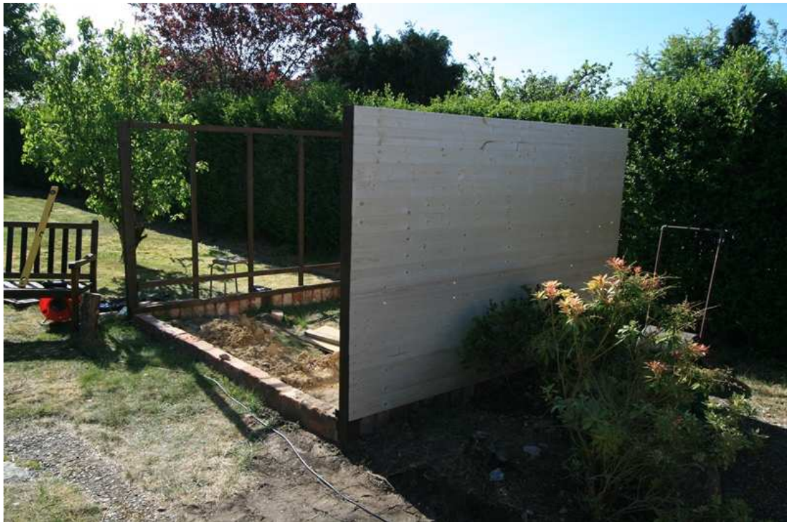
Figure 18 – Screw Shiplap cladding to the frame
