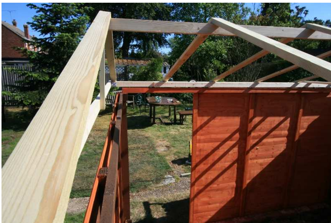
Figure 46 – Roof placed into position (2) – note end overlap
