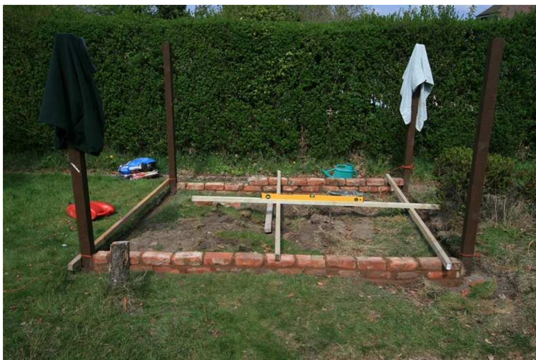
Figure 14 – Checking everything is square and level
