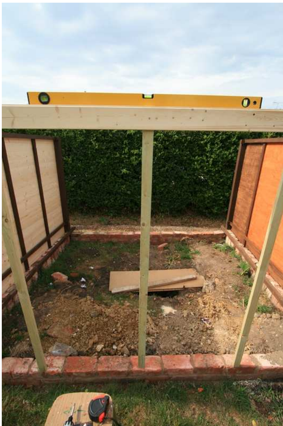
Figure 24 – Ensure roof runner is level
