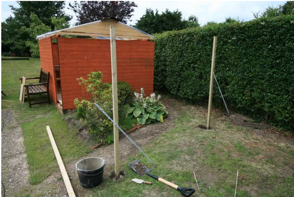
Figure 73 – Add roof runner support posts
