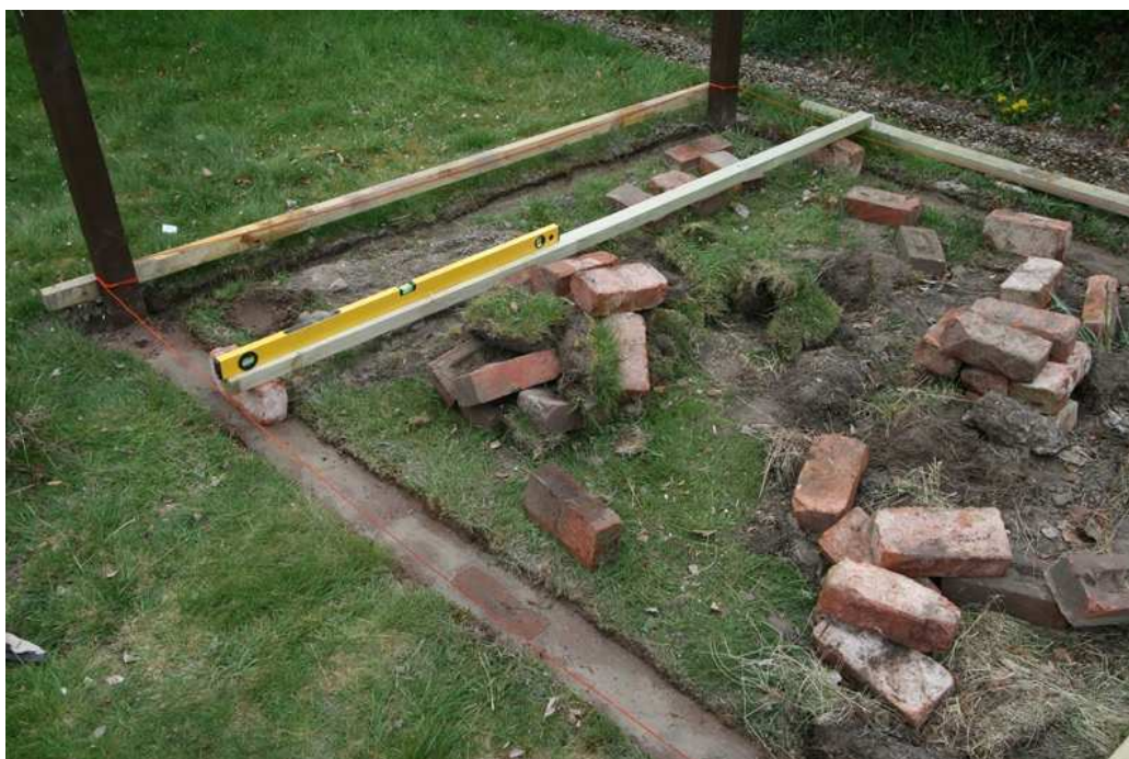
Figure 11 – Concreting done - make certain foundations are square and level
