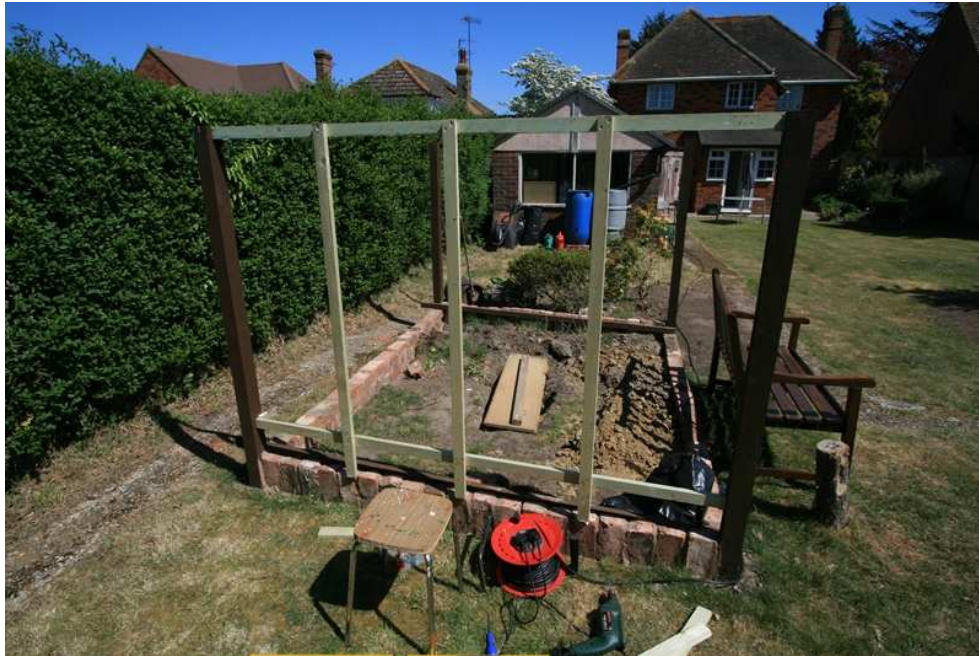
Figure 16 – Start Side Frames
