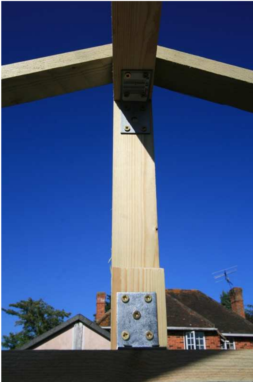
Figure 51 – Adding roof cross braces and brackets (1)
