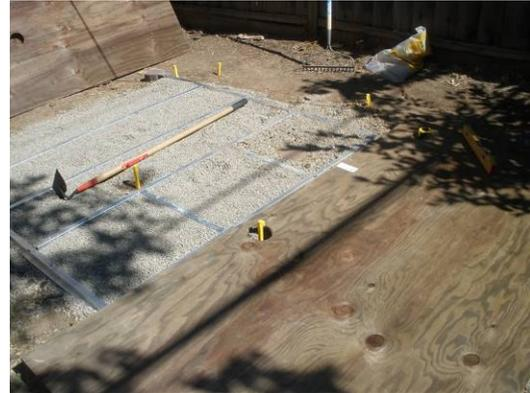
*The stake located in the hole in the floor shows where the bricks should be placed*
