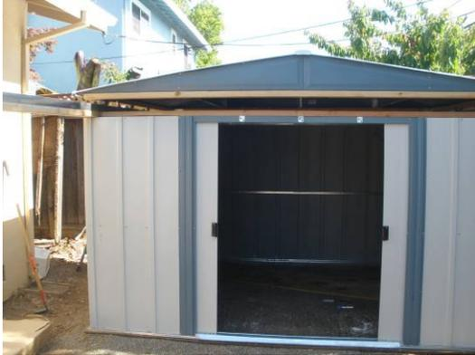
*Complete shed with the gap between the roof and the walls*
