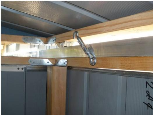
*Turnbuckles keep the roof in place*
